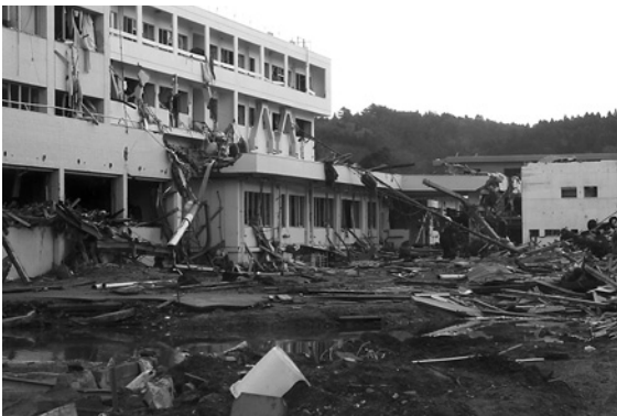
Fig. 1 Shizugawa Municipal Hospital
